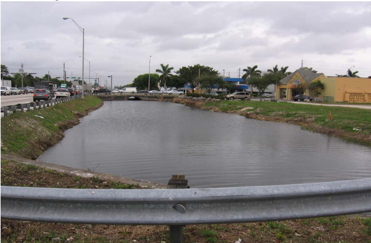
Photograph 2: (NORTHLINE CANAL) North side of NW 25 th St at intersection with NW 78 th Ave, facing west. Shows canal banks with gentle slopes and little erosion.
