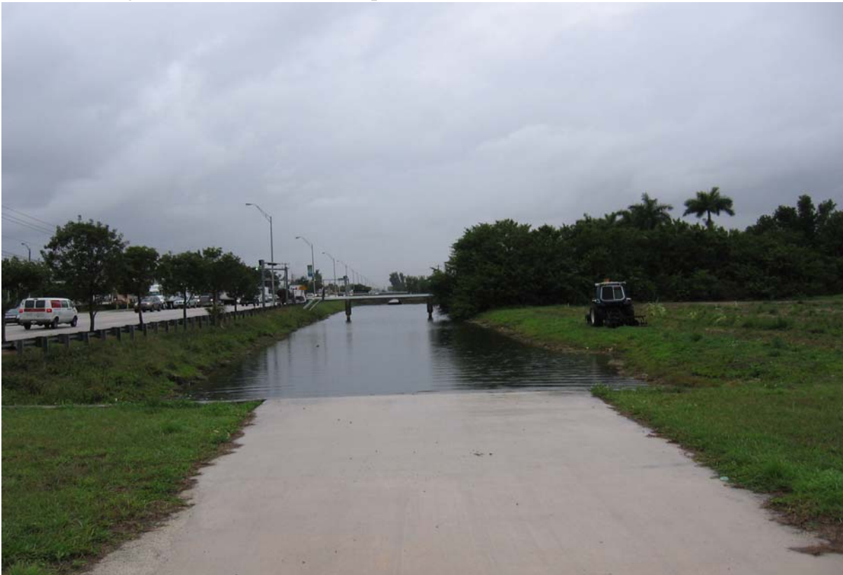
Photograph 6: (NORTHLINE CANAL) North side of NW 25 th St at intersection with NW 27 th St, facing west. Shows canal banks with moderate slopes and little erosion.
