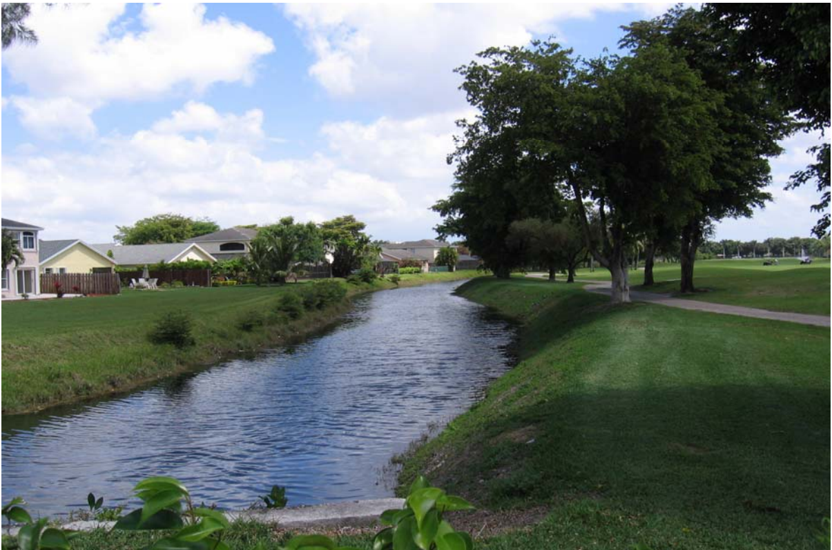
Photograph 28: (DRESSELS CANAL) Canal crossing at NW 102 nd Ave, facing east. Showing moderate to steep grass-covered slopes with little erosion.
