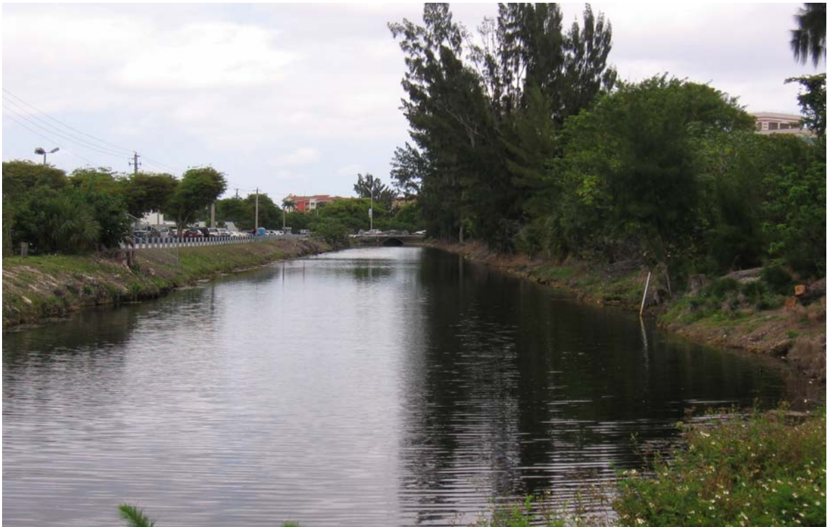
Photograph 34: (DRESSELS CANAL) Canal section just south of Federal Reserve (Doral Blvd), facing northeast. Showing moderate slopes and little erosion.
