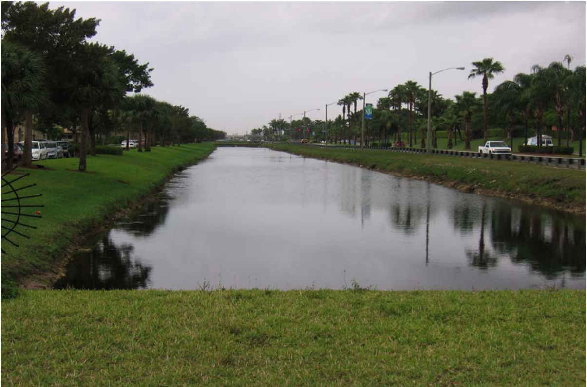
Photograph 21: (DRESSELS CANAL) NW 109 th Ave at intersection with NW 58 th St, facing west. Shows canal banks with gentle to moderate slopes and little to moderate erosion.
