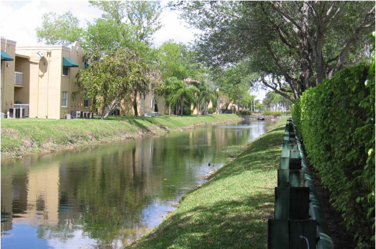
Photograph 29: (DRESSELS CANAL) West side of NW 97 th Ave just south of NW 49 th Ter, facing north. Showing moderate grass-covered slopes with little erosion.
