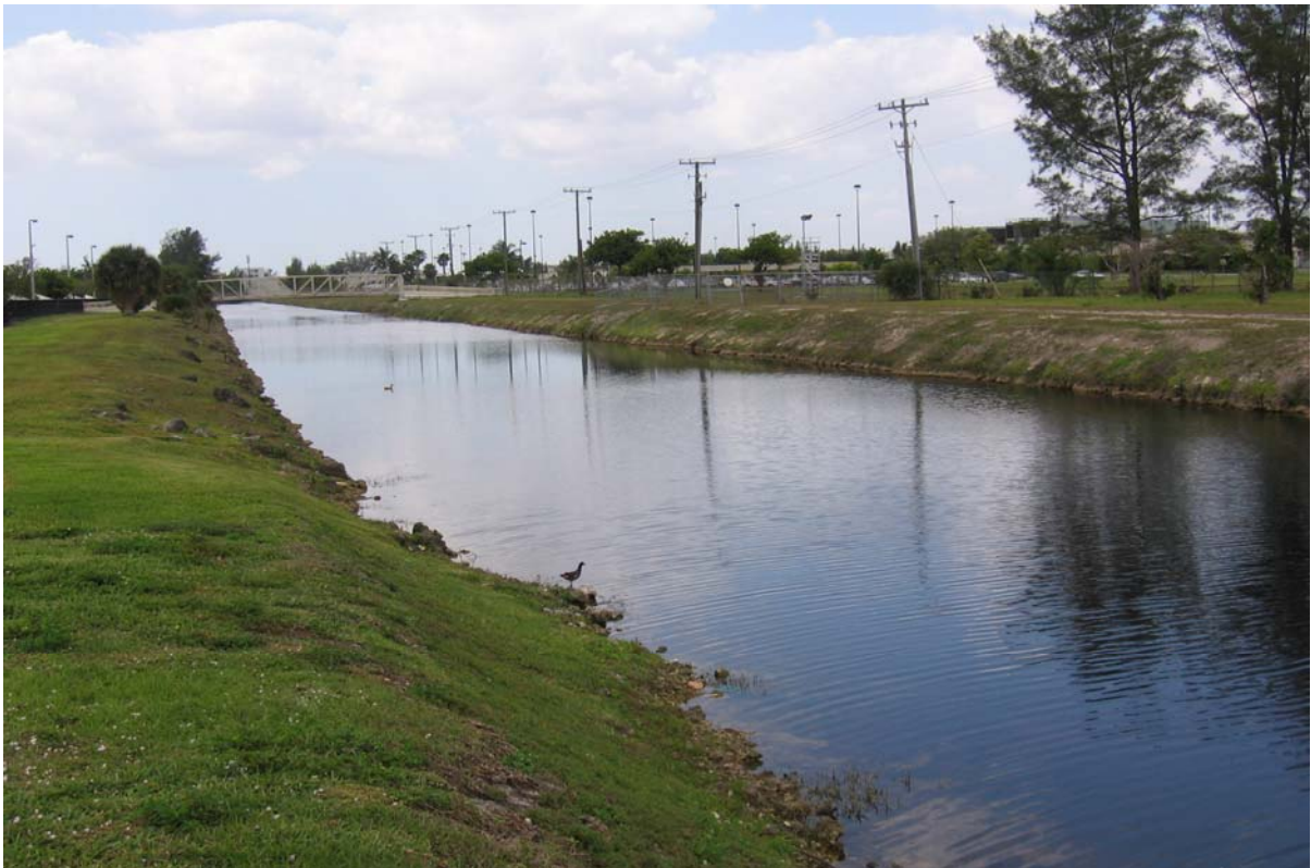
Photograph 33: (DRESSELS CANAL) Canal section just south of Federal Reserve (Doral Blvd), facing west. Showing moderate slopes and little erosion. Numerous boulders visible along south bank.
