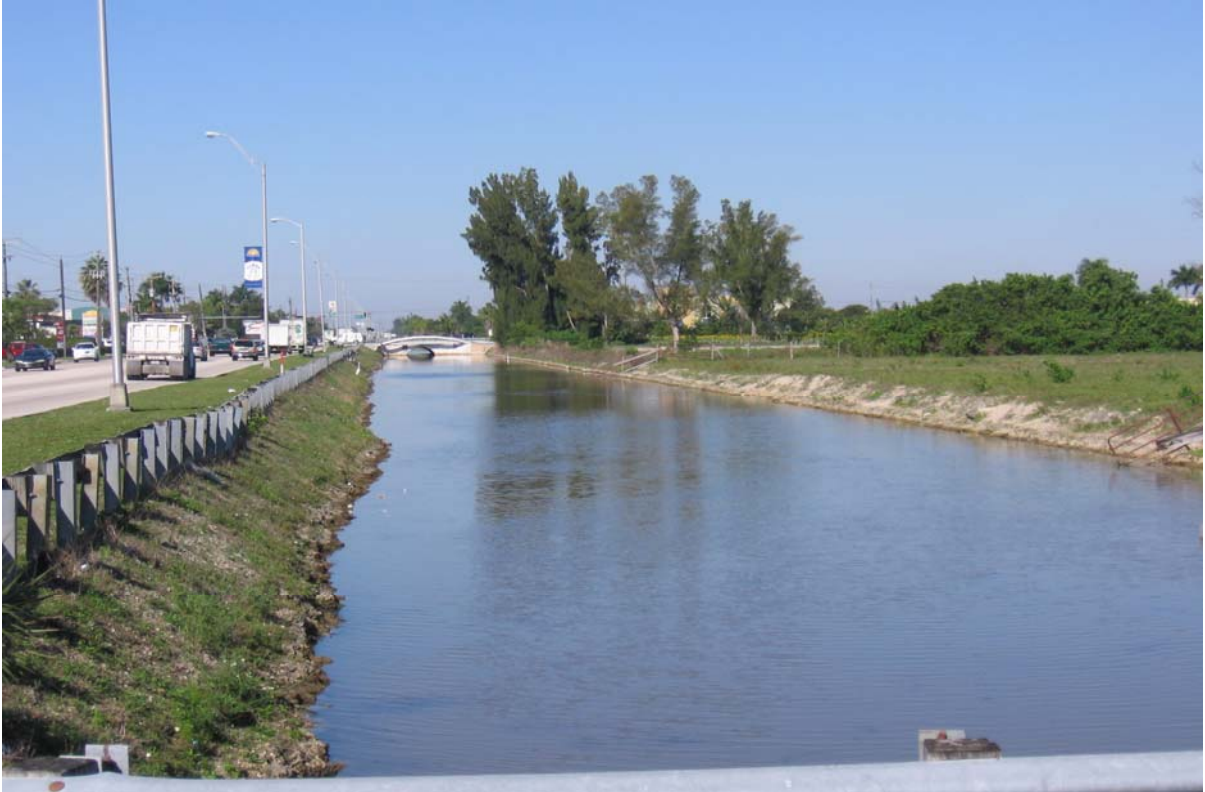
Photograph 8: (NORTHLINE CANAL) North side of NW 25 th St at intersection with NW 94 th Ave, facing west. Shows canal banks with moderate slopes and little erosion.
