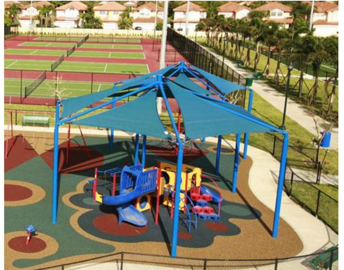
**Key Consideration is Removing Shading For A Storm Event**
