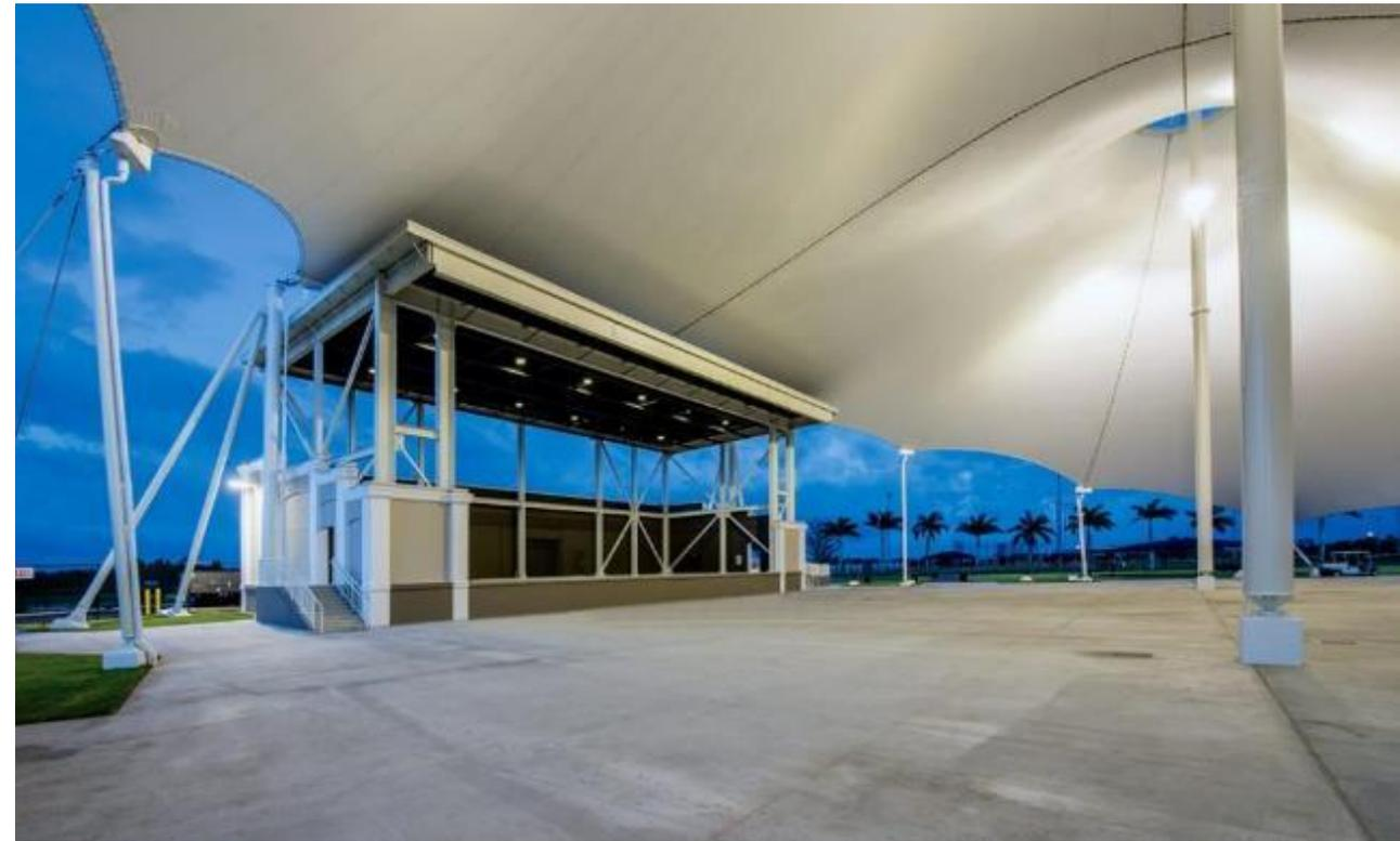
Sound and lights are attached to stage system separate from tensile structure
