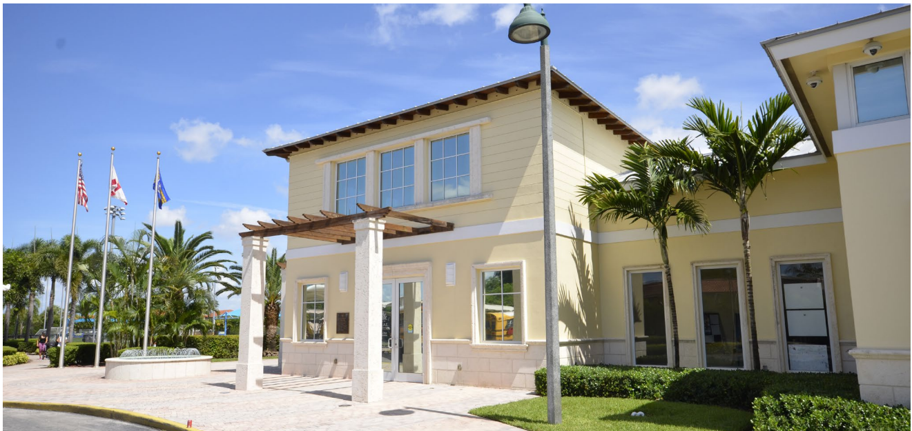
Figure 5.2: Morgan Levy Community Center that is recommended for future expansion to 15,000 SF.
