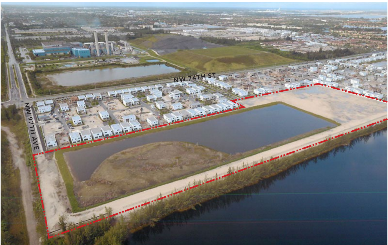
Figure 2.59: Aerial photograph taken during construction, indicating the location of Doral Glades Park (City of Doral, 2016b).
