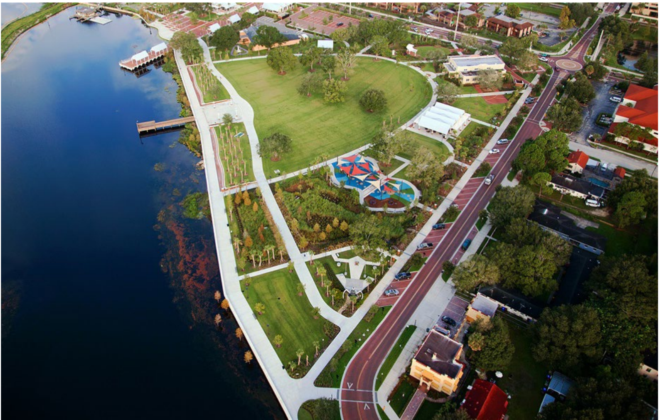
Figure 4.11: Kissimmee Lakefront Park in Central Florida (Burkhardt Construction, Inc., 2018).
