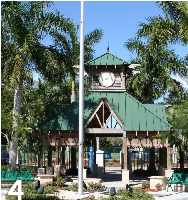
Figure 2.55: Gateway pavilion at the entrance of the park.
