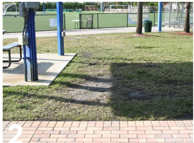
Figure 2.42: Example of wear and tear present near the soccer fields.
