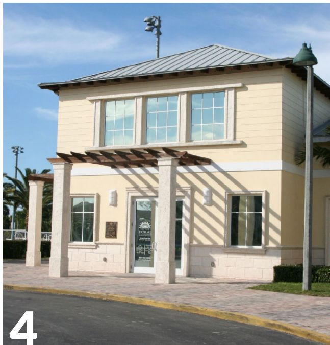
Figure 2.45: Morgan Levy Park Community Center entrance.
