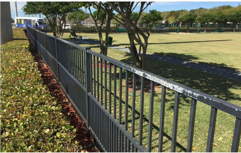
Figure 4.22: Example of the deteriorating finish of the aluminum fencing at Trails and Tails Park (2016).
